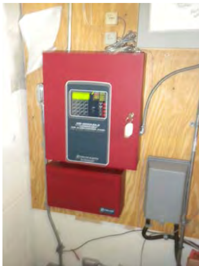
View of the central fire alarm control panel
