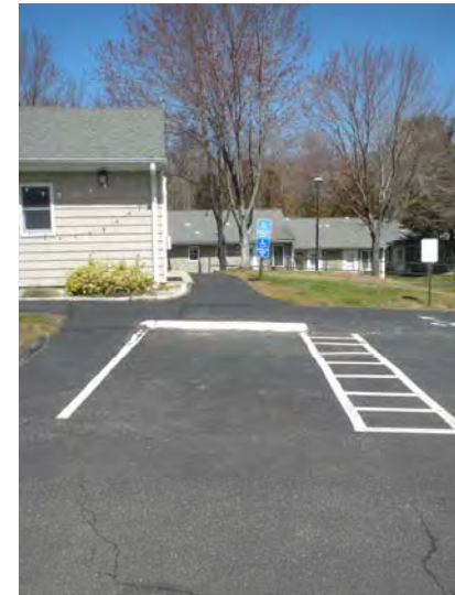
Handicapped parking space lacking compliant access aisles
