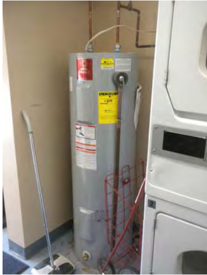
View of the laundry room domestic hot water tank
