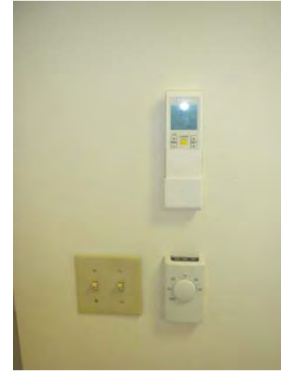
Thermostat and heat pump control
